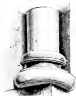
Base of niche shaft.
